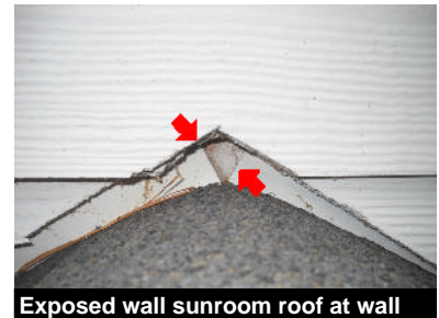
Exposed wall sunroom roof at wall
