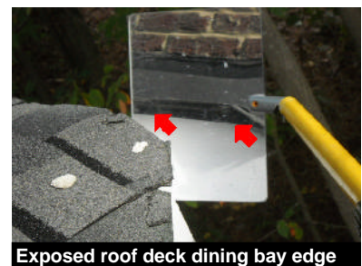
Exposed roof deck dining bay edge
